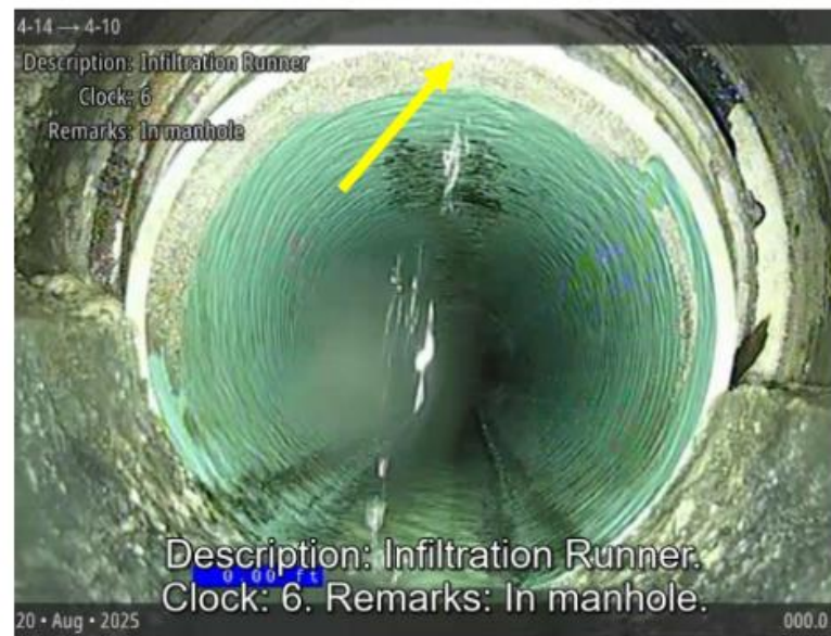
Manhole 4-14 (Fishman Road)
