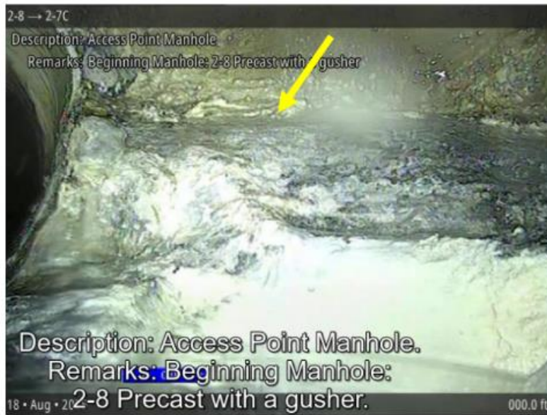
Manhole 2-8 (S. Lakeshore Drive)
